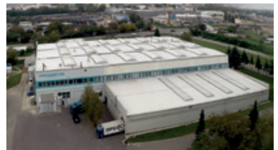
Production plant and logistics centre in Znojmo (Czech Republic)
